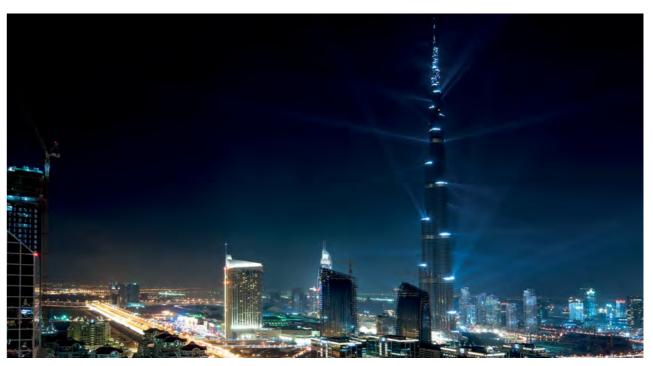
Burj Kalifa, the tallest tower till date standing at 828 meters high. Master Builders Solutions developed a concrete mix that can be pumped to a height of >600 meters without interruption, to shape the structural form of the tower. Withstanding high ambient temperatures without segregating, MasterGlenium Sky admixtures
