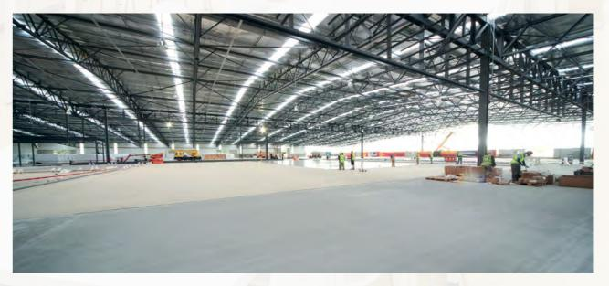
Commonly known as 'Project Century', Lion Nathan brewery situated in South Auckland is built to last for 100 years. Constructed with a focus on quality and longevity, floors for the facility were installed with Ucrete DP heavy duty PU-hybrid system to meet the performance expectations.
