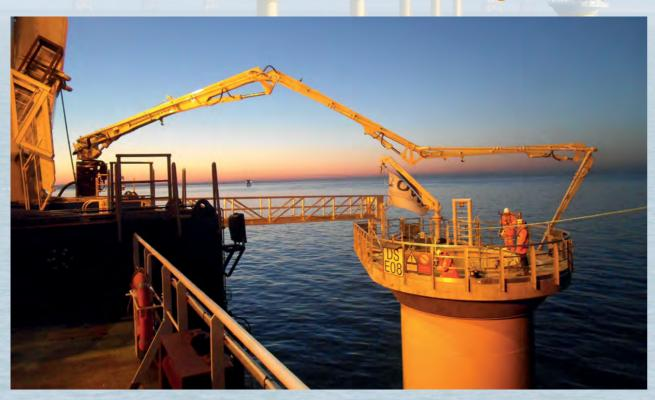
MasterFlow 9500 Exagrout was pumped into the monopile transition piece connections using the FoundOcean Super Pan Mixer. The project to install 108 foundations is a world record in the industry, and a new benchmark for future offshore windfarms.
