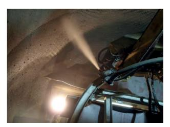
Construction of the world's longest rail tunnel - a 57 kilometer Gotthard Base Tunnel. Combining MasterGlenium superplasticizers - to make the concrete flowable and workable, with shotcrete accelerators - to allow concrete to solidify and harden within seconds after being sprayed on the tunnel wall.
